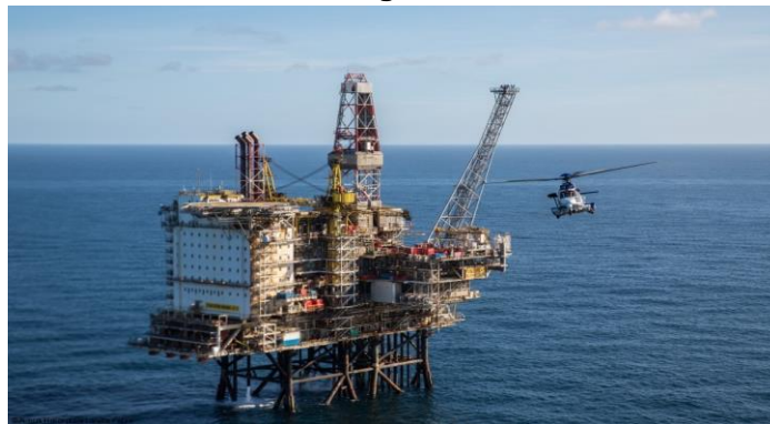
Oil and gas facilities
